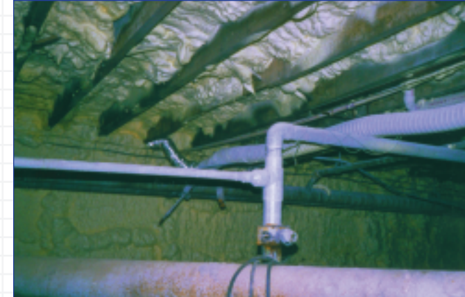
After 3.0 inches of Icynene® was applied underneath the floors and on the walls of the crawlspaces
