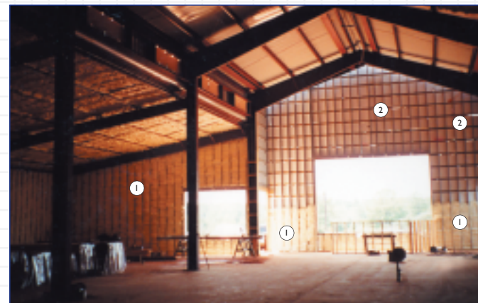
Icynene® installed into the exterior wall cavities, prior to the installation of drywall. (1) Icynene® sprayed area, (2) unsprayed area, note the gaps where air can freely pass through the wall. Daylight highlights these gaps.
