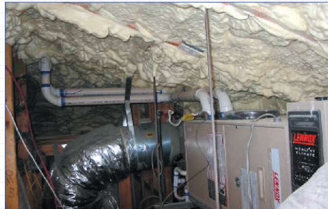
Icynene was sprayed on the underside of the roof deck to seal the building and convert the attic from unconditioned to conditioned space, thereby increasing the efficiency of the heating and cooling system.
