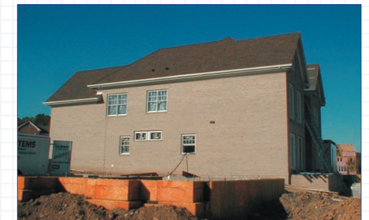
Icynene® is installed by an Icynene Licensed Dealer to facilitate the construction process, allowing the builder to build a durable, airtight envelope with less sealing material.
