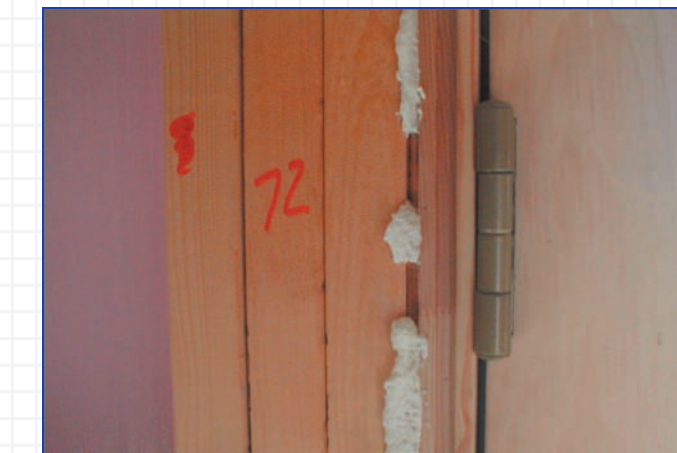
Icynene® softly expands to 100 times its initial volume to completely fill all gaps and crevices that compromise airtightness.
