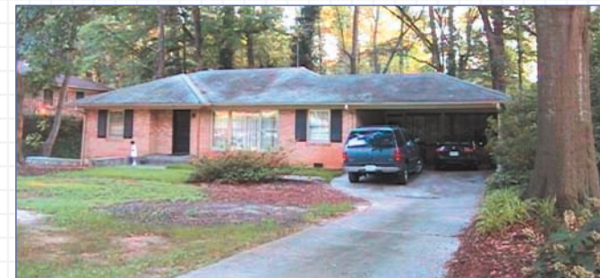
The Cartledge residence in Atlanta, GA was a classic 1950's style ranch. The renovation increased the size of the house to 4,921 sq. ft. from 3,338 sq. ft.
