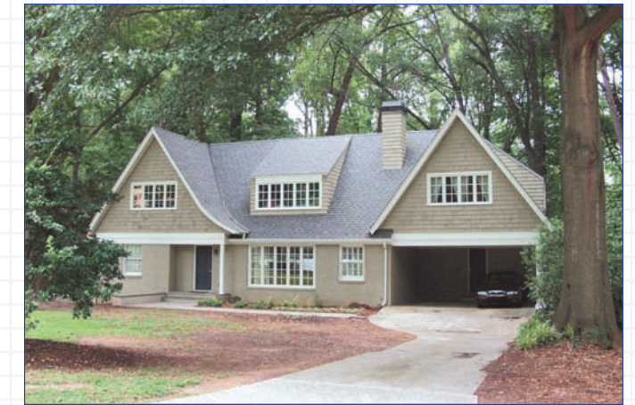
The Icynene®-insulated home surpassed all of the EarthCraft House™ guidelines. The Cartledges were able to decrease their heating and cooling consumption by 12% and 54% respectively.
