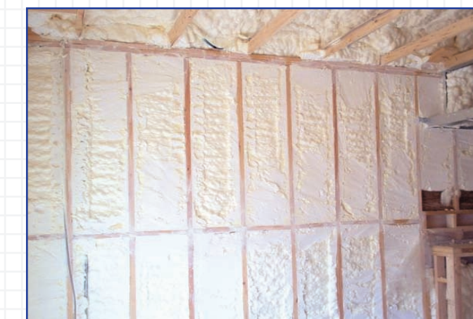
With Icynene® sprayed into the exterior wall cavities, the sound from the quarry 2 miles away will be minimized, thereby ensuring the comfort of the residents and staff of the Home.
