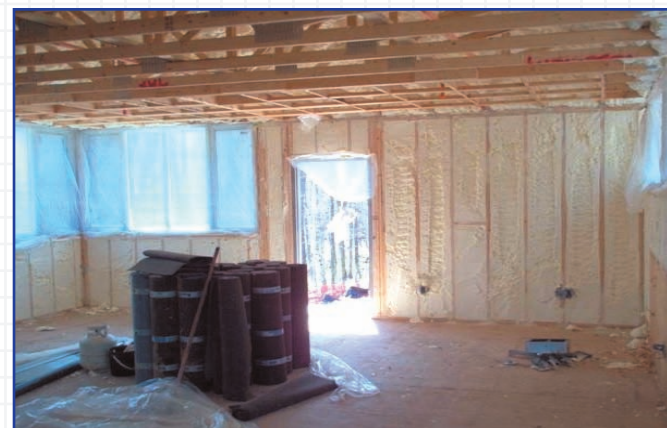
Icynene® was so effective at minimizing air transport that it eliminated the need for additional sealing material.
