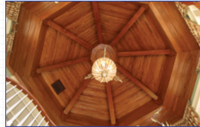
Decorative wood strip was applied with no problems because Icynene® effortlessly adheres to the cavity. Photo courtesy of IBACOS, Inc. (www.ibacos.com)
